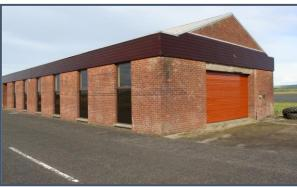
Constructed in the 1970s for operational office and storage use, this brick, built, single-storey structure has a pitched profile metal clad roof over a timber frame and concrete floor.
